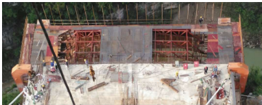
(b)底篮拼装实物照片
