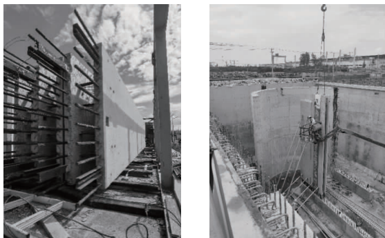
(a)叠合墙现场堆放 (b)叠合墙临时支撑及安装
