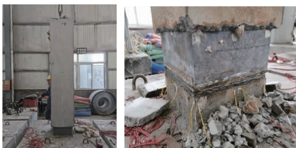
(a)墩柱吊装对接 (b)上下连接钢管焊接
