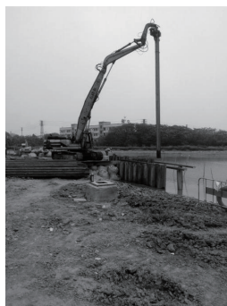
(a)施打钢板桩
