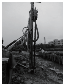
(b)袖阀管注浆
