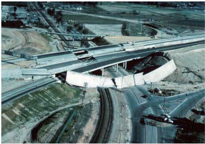
图1 San Fernando地震中破坏桥梁
